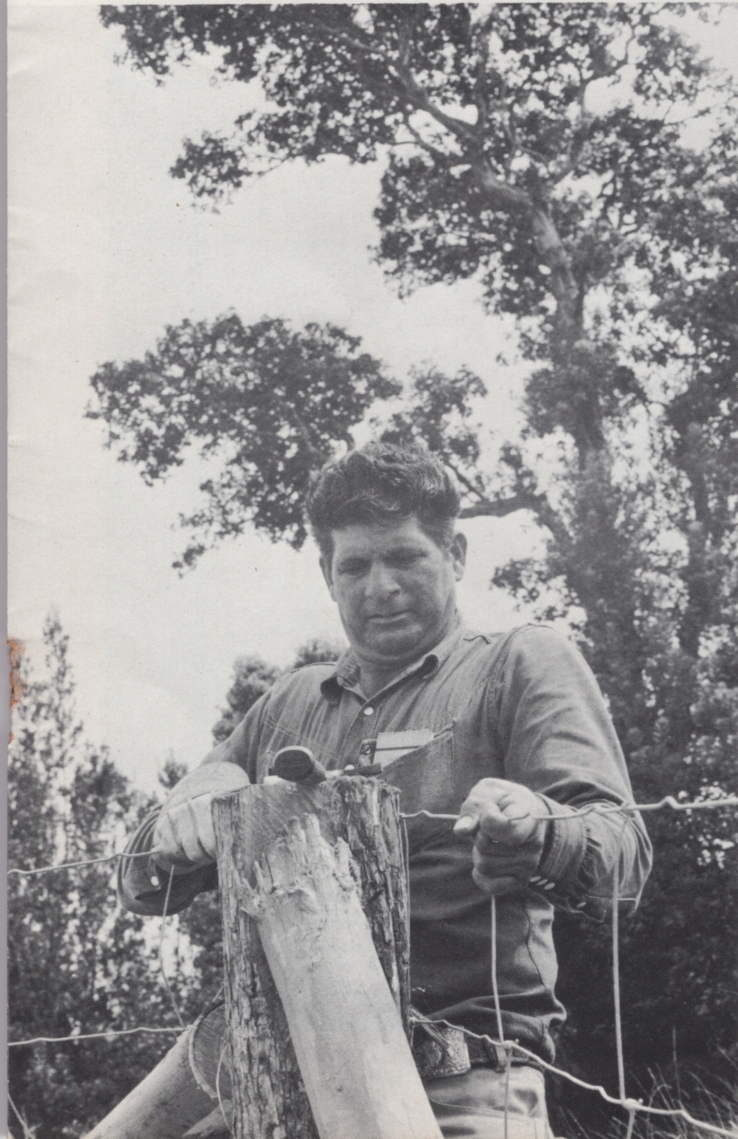
After the fence is stretched out on the ground, it is pulled up against the fenceposts by the truck and the men.
